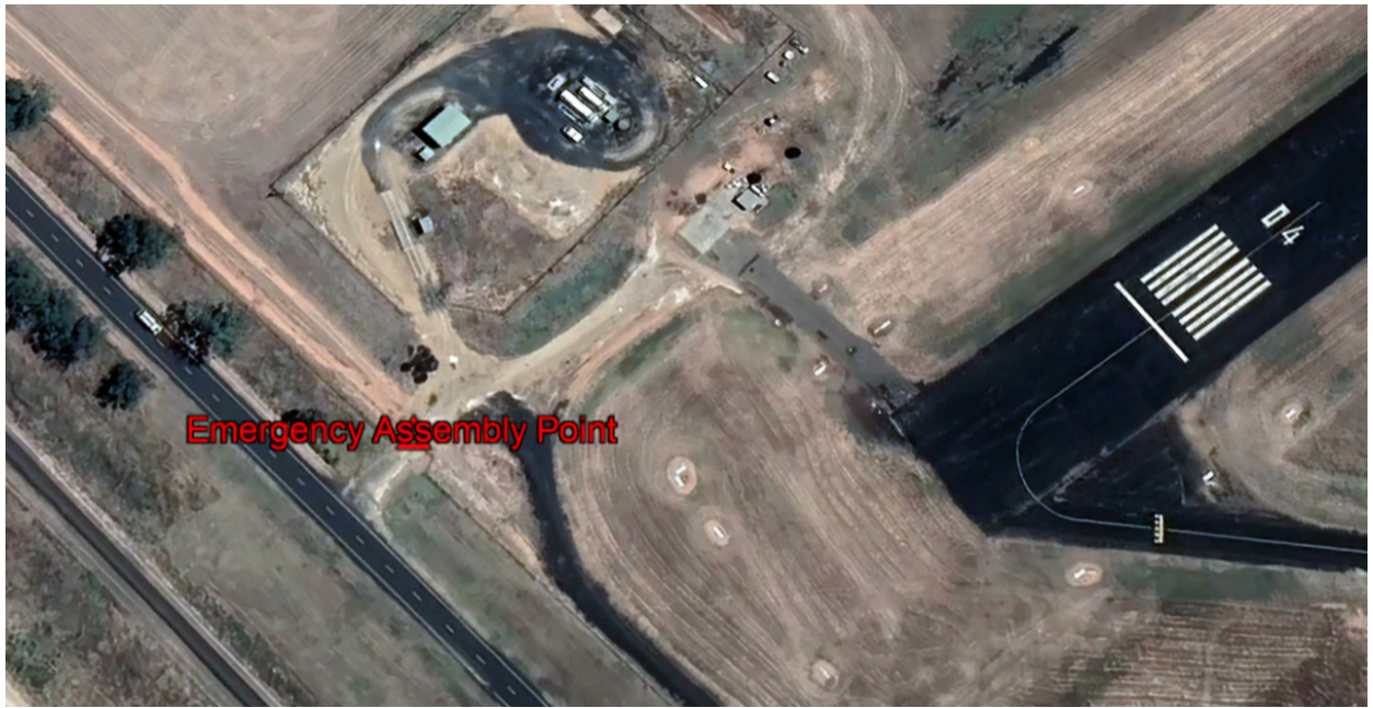
Emergency Assembly Point
