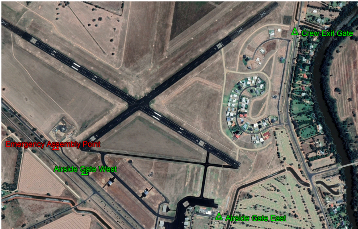
Airfield Access Gates
